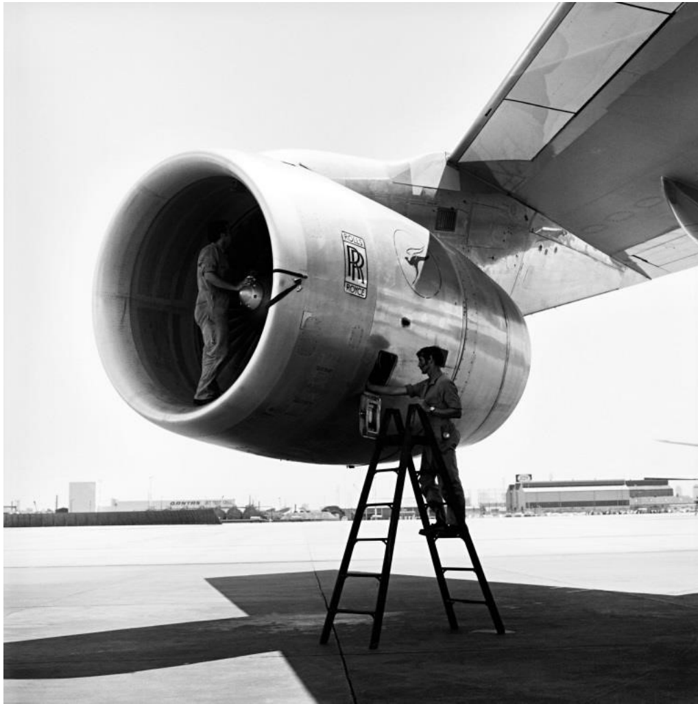
No 22 - 747-38SP VH-EAA – Rolls Royce RB211-524B2 Engine
